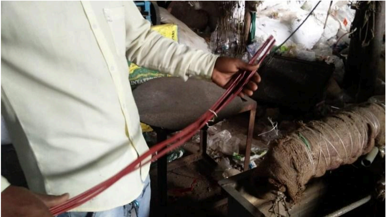
Figure 11. Cables of plastic
